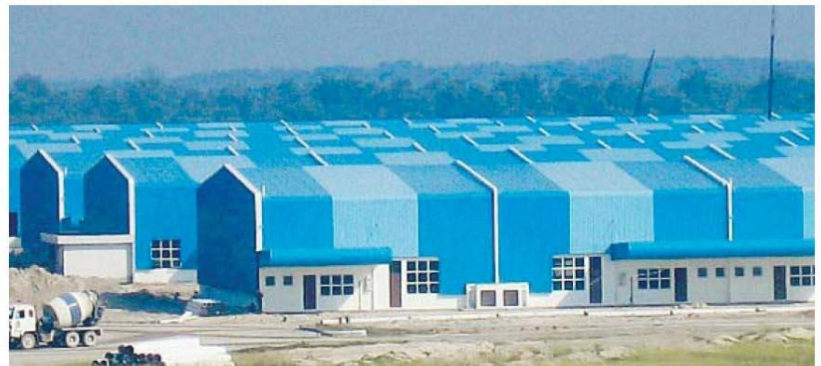
The completed light industrial units at the Port Klang Free Zone in Pulau Indah which will spur industrial growth.
