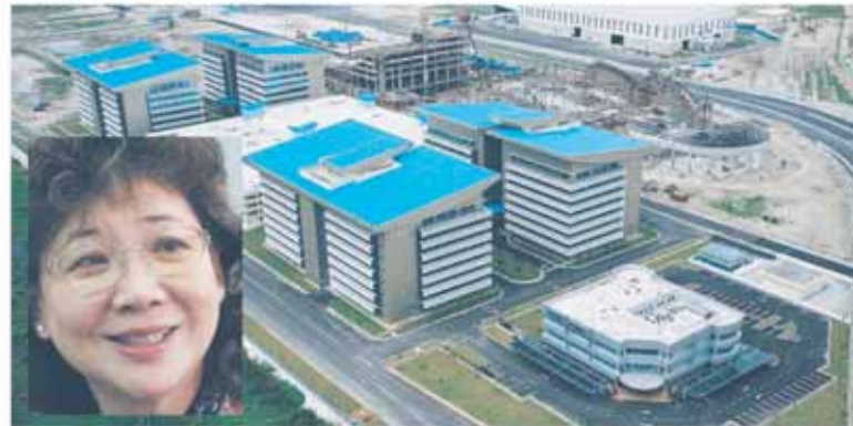
An aerial view of the Port Klang Free Zone. Inset is Datin Paduka O.C. Phang
